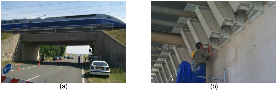
Figure 1 – PK 075+317 bridge on the Paris-Lyon high speed track and strengthening system
