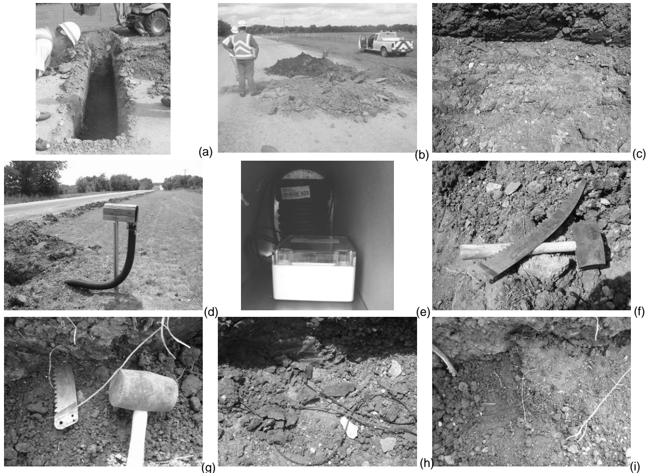
Figure 8. Moisture sensor installation procedures: (a) Trenching; (b) Separation of base and subgrade; (c) Leveling of installation site; (d) Protective tubing and datalogger containment system; (e) Datalogger; (f) Tools for pre-insertion of sensor; (g) Pre-insertion; (h) Installed sensor; (i) Compaction near sensor head
