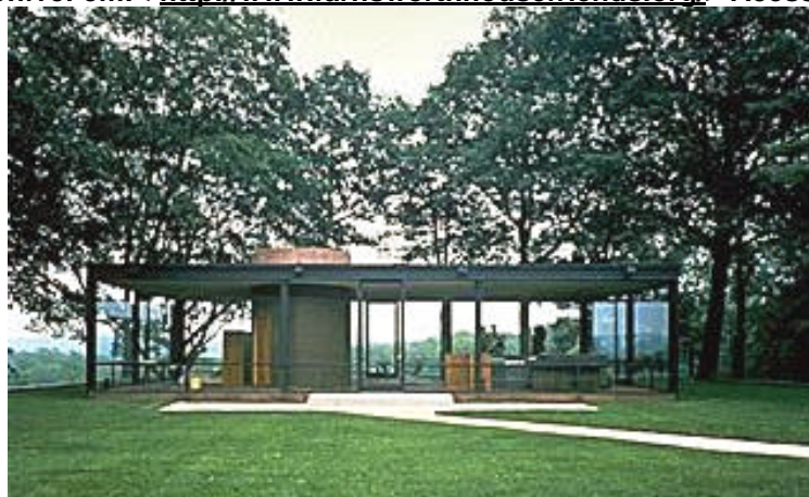
Figura 1.3 – Vista frontal Glass House.
