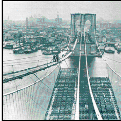
Figure 7: Construction of the Brooklyn Bridge Source: Museum of New York 10
